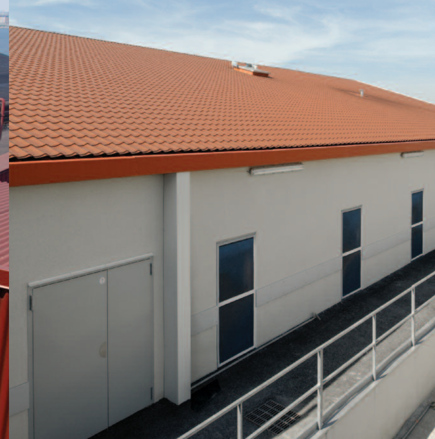
Project: LIDL Supermarket, ZA de la Mirandole, Villerest, France Architect: © Albert Mathieu, Bureau d'études ALBERT, 57 Building system provided by: BACACIER Photography: © Nicolas Fussler
