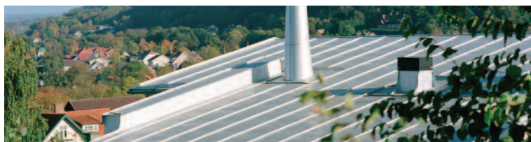
Project: Private housing Photographer: © LINDAB Buildings
