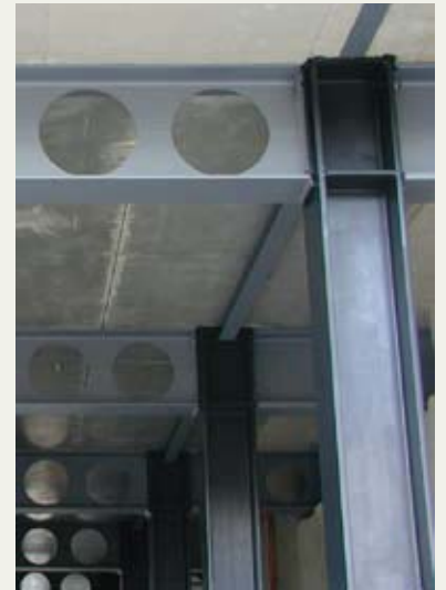
Figure 17: Assemblage poutre-poteau
