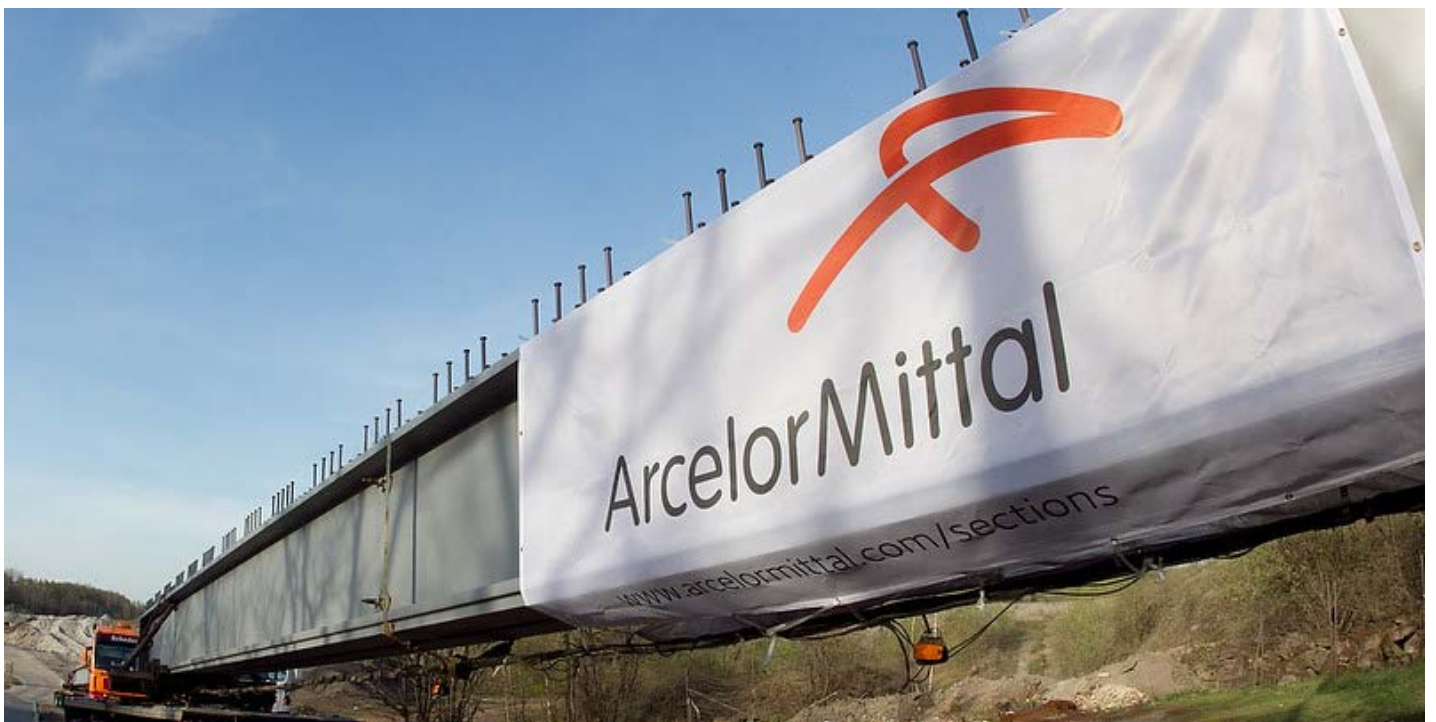
Delivery of a 41.7 m fully finished heavy section to the construction site of a bridge for 86N express way in Bernburg, Germany
