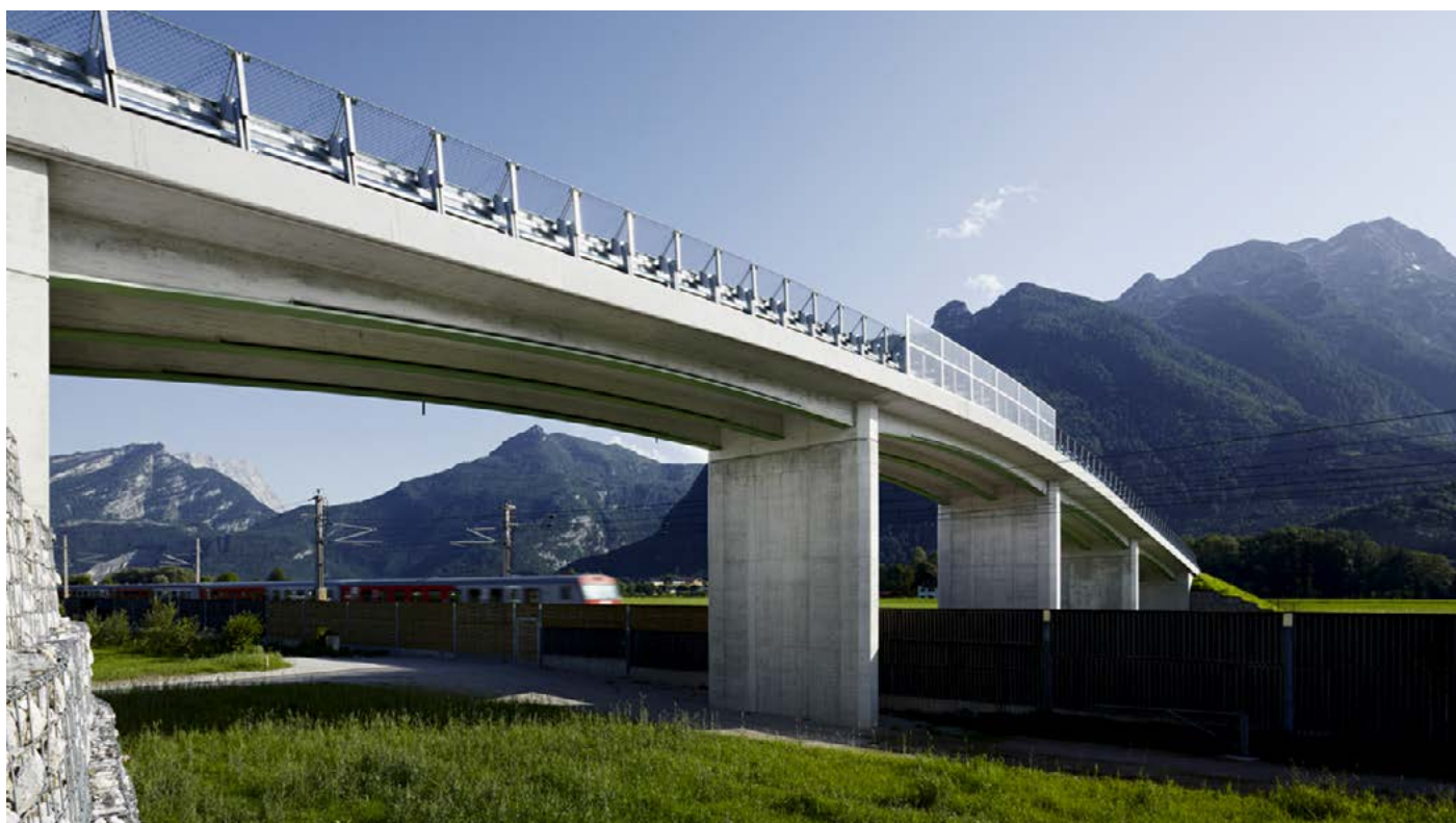
Overpass on ÖBB line, Kratzerau, Austria (©: SSF Ingenieure)
