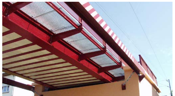
Half-through bridge deck in Guenange, France
