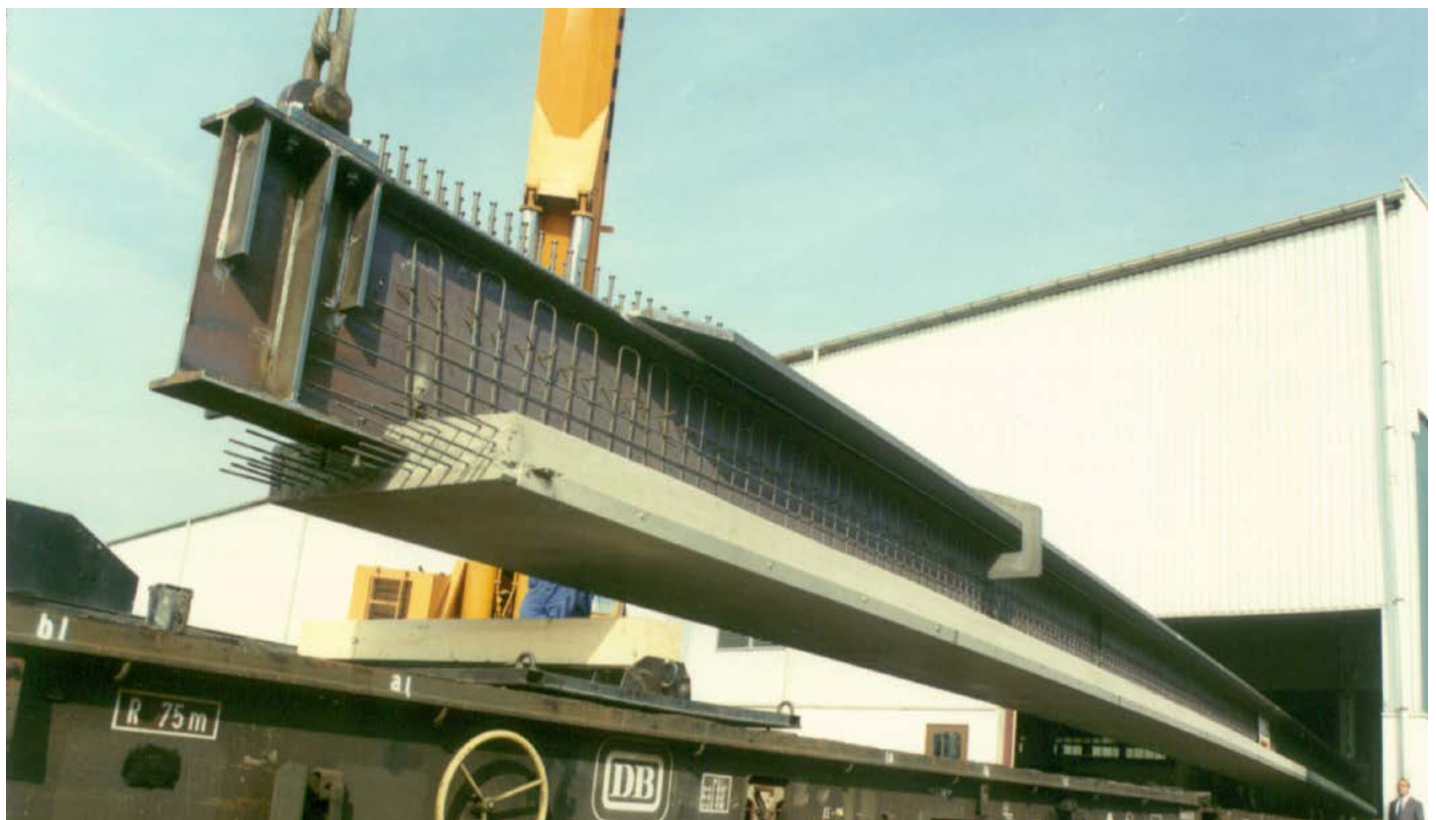
Preflex girder for bridge in Kerpen Horren, Germany
