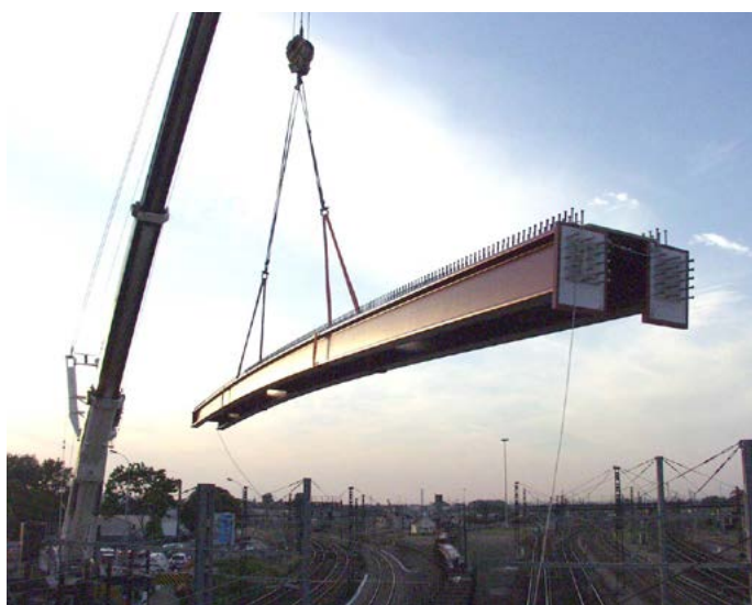
Choisy bridge, Villeneuve-Saint-Georges, France
