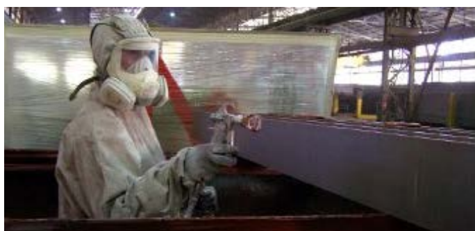
Manual application of an organic layer
