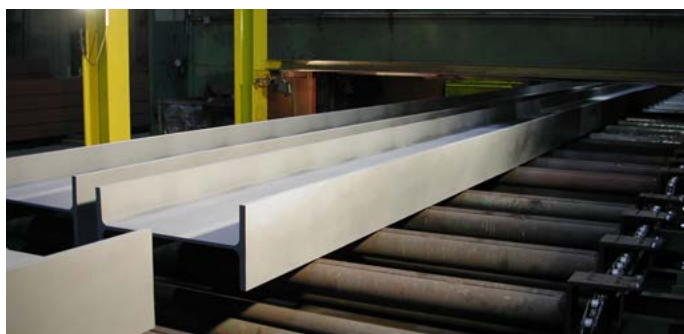
Automatic shot blasting to grades Sa 2.5 or Sa 3.0 and application of shopprimer
