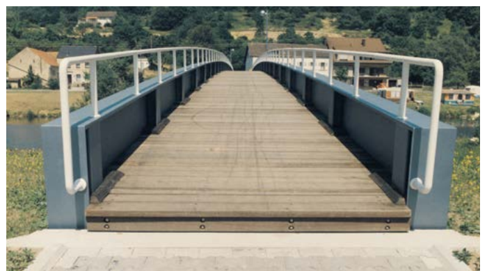
Footbridge in Steinheim, Germany
