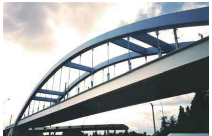
This example shows a bow-string bridge for the Mediterranean high speed railway line over the French highway A7 near Avignon (F). A filler beam deck has been used to span transversally to the bridge axis.
