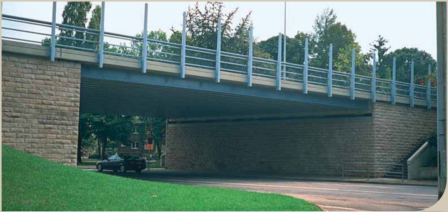
Filler beam deck bridge in Esch-sur-Alzette, Luxembourg - 19 m span; 0.65 m deck depth. For aesthetic reasons the edge beams are not encased in concrete on the outer side.
