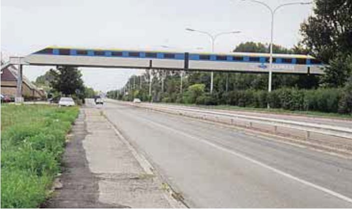
Footbridge for the visitors of a leisure park in Wavre, Belgium – Through type bridge with thematic enclosure.
