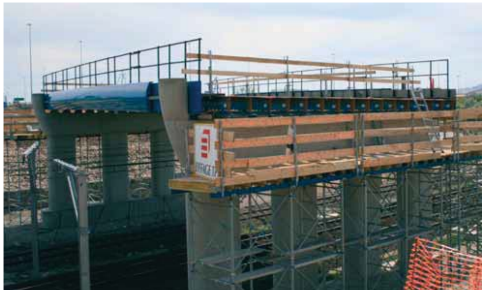
Assembled first span over the existing railway line.
