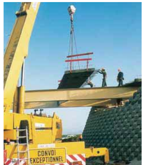
Prefabricated slab – erection of a precast concrete element.
