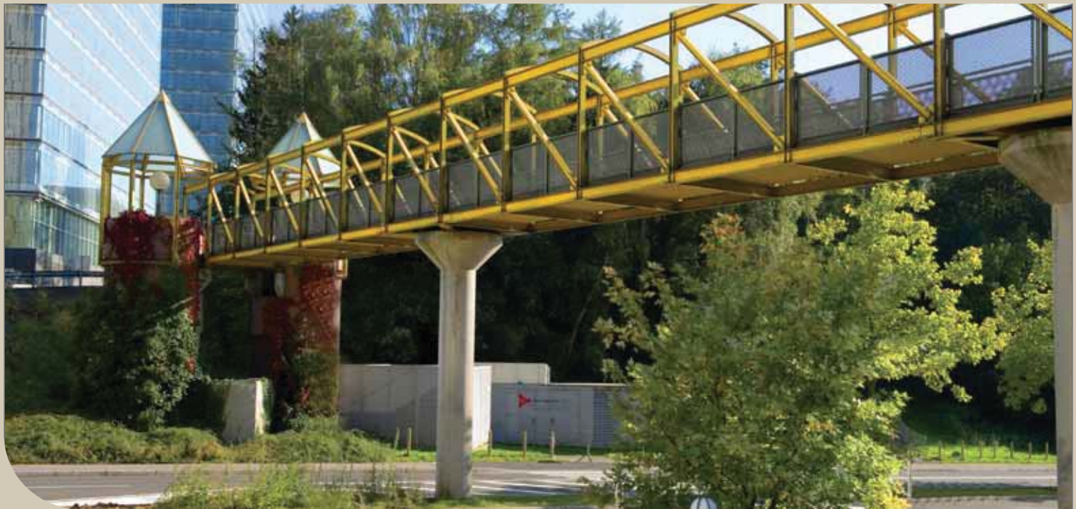
Access footbridge to the building of the Court of Justice of the European Communities, Luxembourg – Architectural design based on lattice girders.
