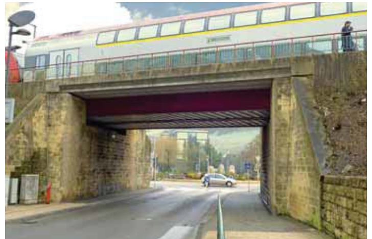
Reconstruction of the railway bridge over EmileMark street in Differdange, Luxembourg - Because of the very restricted construction depth, two single track half-through type bridges were implemented.
