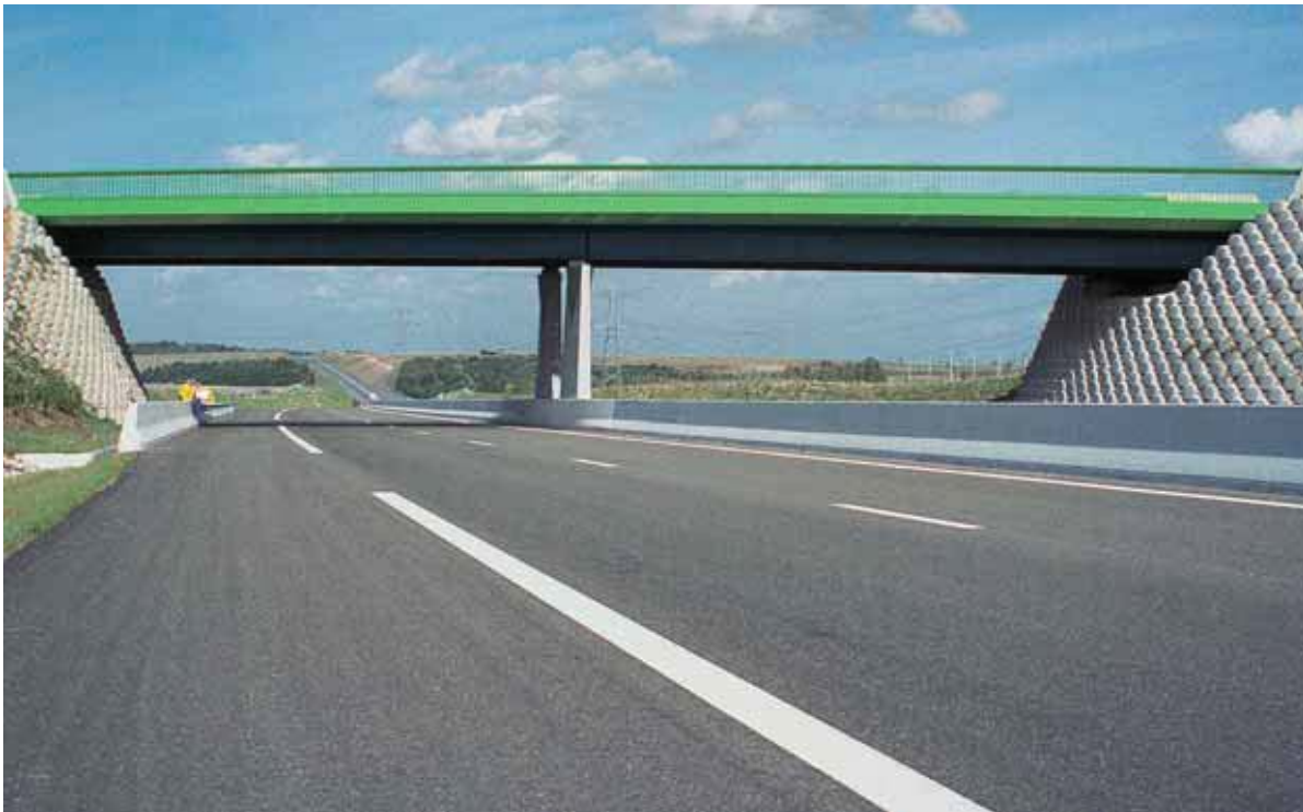
Road bridge over the A16 motorway, France - Composite deck with two main girders in high strength steel S 460 M.
