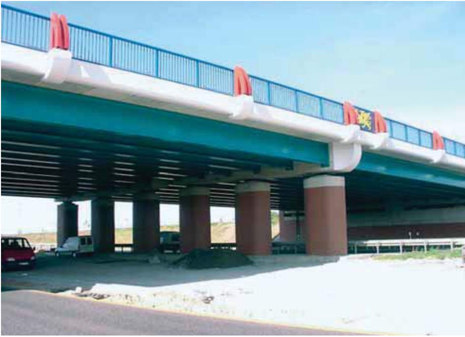
Composite bridge with concrete crossbeams at Bentwisch, Germany – Design combining steel and colour.
