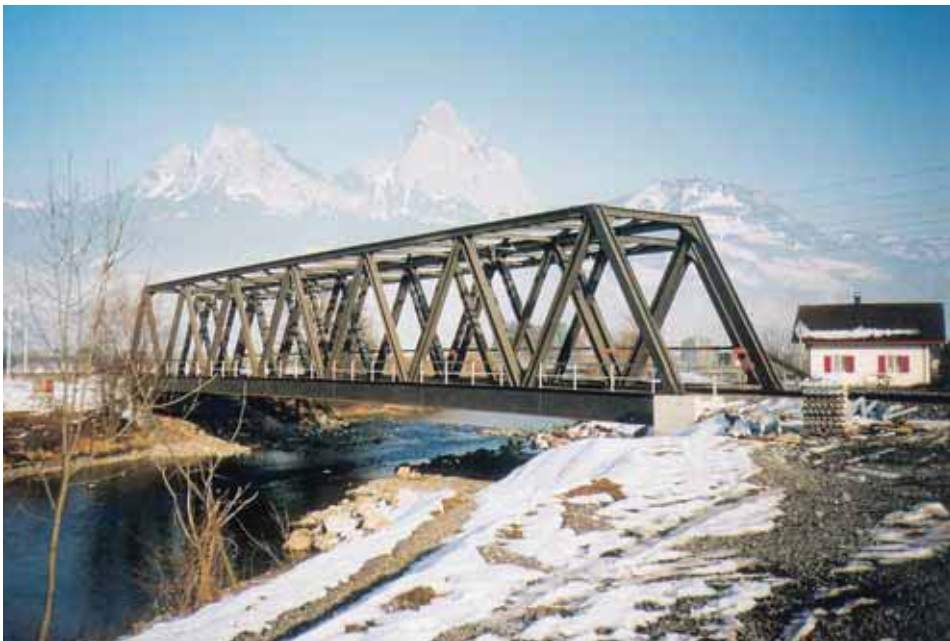
Reconstruction of the bridges over the Muota river, Gotthard -line of the Swiss Federal Railway Company - Diagonals and upper chords are made of rolled beams (HD and HE shapes). Thermomechanically rolled steel was used for enhanced weldability.
