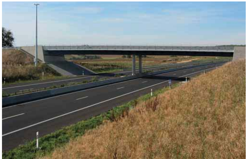
Bridge link with two spans of 23.9 m to La Sarre, Luxembourg – The composite bridge is a twin-girder bridge with box sections of two longitudinally welded rolled beams.
