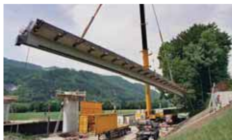
Lifting-in of a PreCoBeam for the bridge at Vigaun, Austria.
