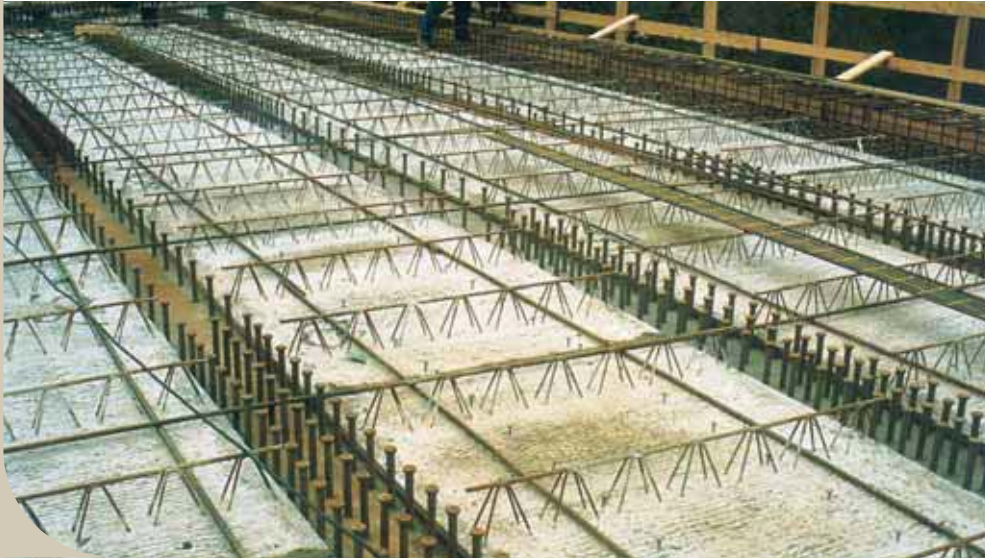
Precast reinforced concrete panels used for permanent formwork.
