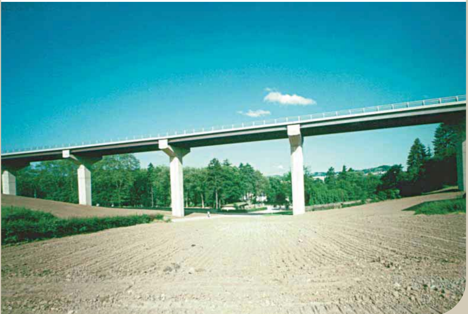
Multiple span viaduct at Ditgesbaach, Luxembourg
