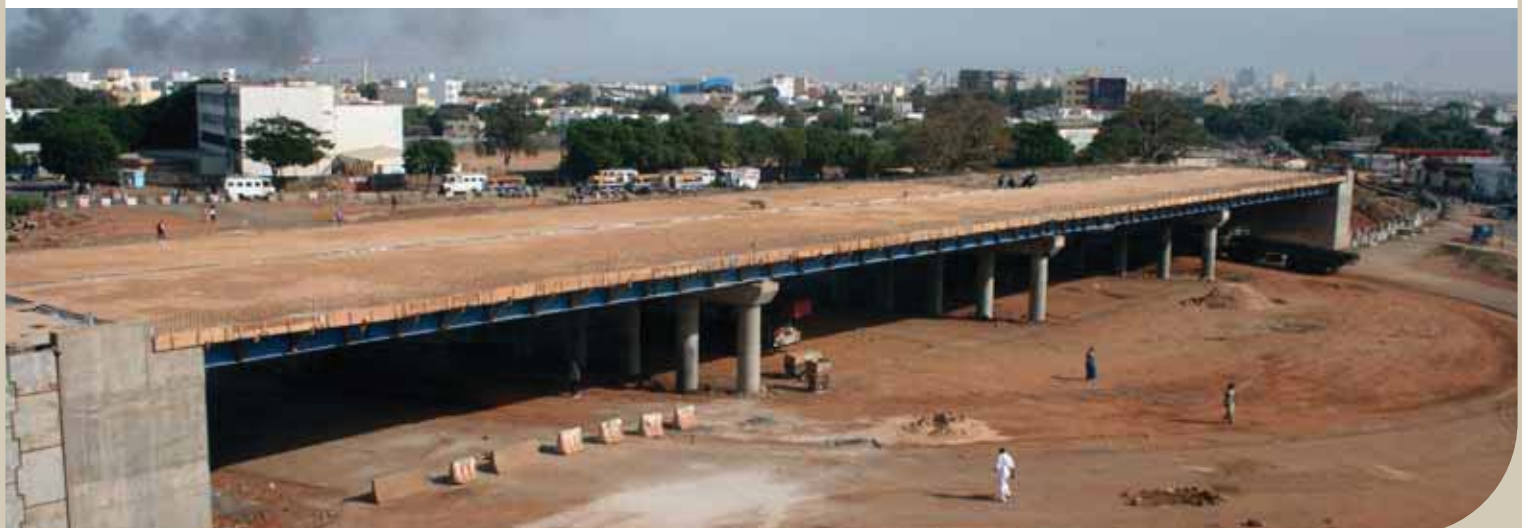
VDN bridge in Dakar, Senegal
