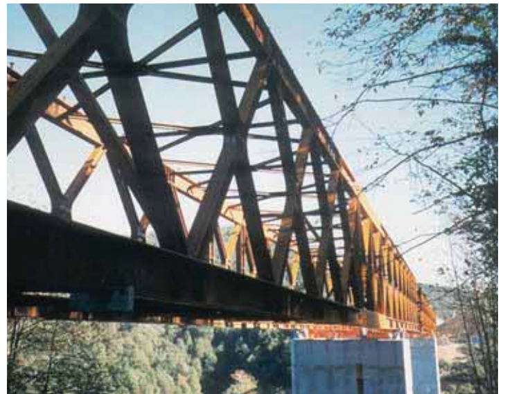
Costa Martina road bridge, Spain – Rolled beam truss girders, continuous over 3 span of 60.6 - 121.2 - 60.6 m. The picture shows the bridge before the erection of the precast slab elements on the upper chords.
