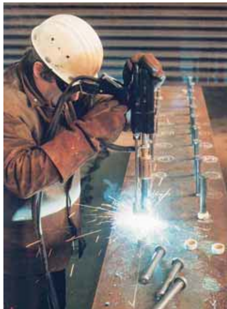
Finishing workshop - Welding of shear stud connectors.
