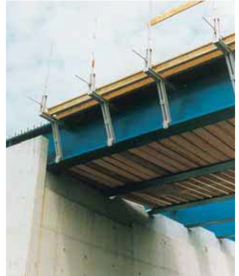
Example of formwork support for cantilever part of slab.
