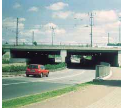
Multiple track railway bridge in Nienburg, Germany - The longitudinal profile of the road and the tracks greatly restrict the available construction depth.
