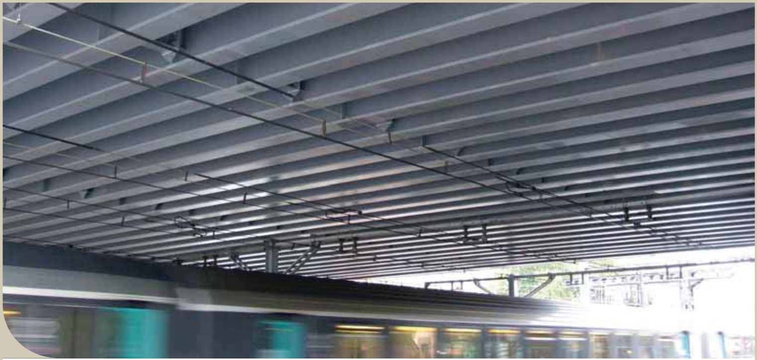
Gosnat bridge in Vitry, France
