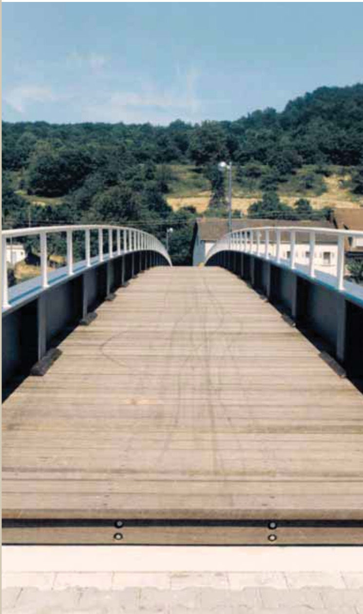
View on the wooden walkway of the half-through bridge with rolled sections in Steinheim, Luxembourg
