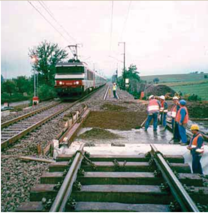
Railway bridge at Berchem, Luxembourg
