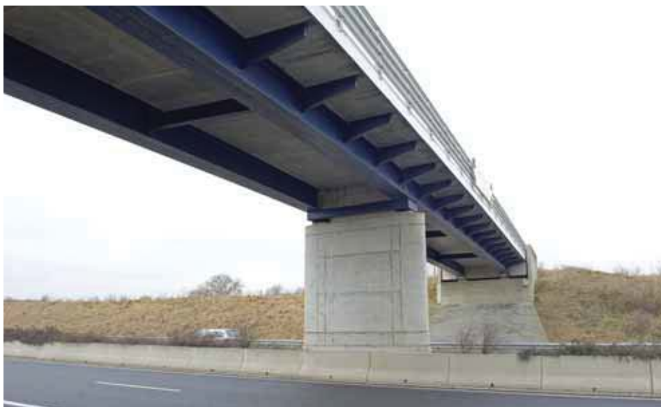
Bridge link to La Sarre, Luxembourg – The large cantilevers have been designed to support the prefabricated concrete elements during construction without any scaffolding, the box sections have been designed to resist the resulting torsional moment.
