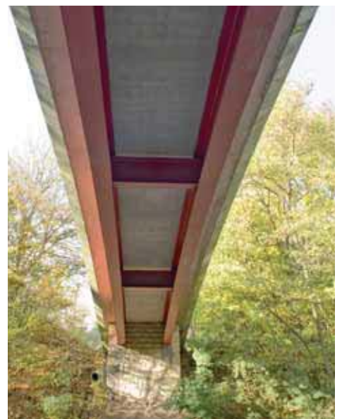
Bottom view on the twin-girder, composite footbridge at Wasserbillig, Luxembourg
