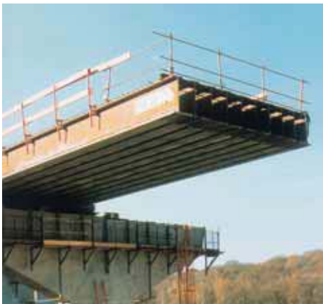
Railway bridge of the TGV Atlantique high speed line in Massy, France – Launching of the beams over the A10 motorway interchange.
