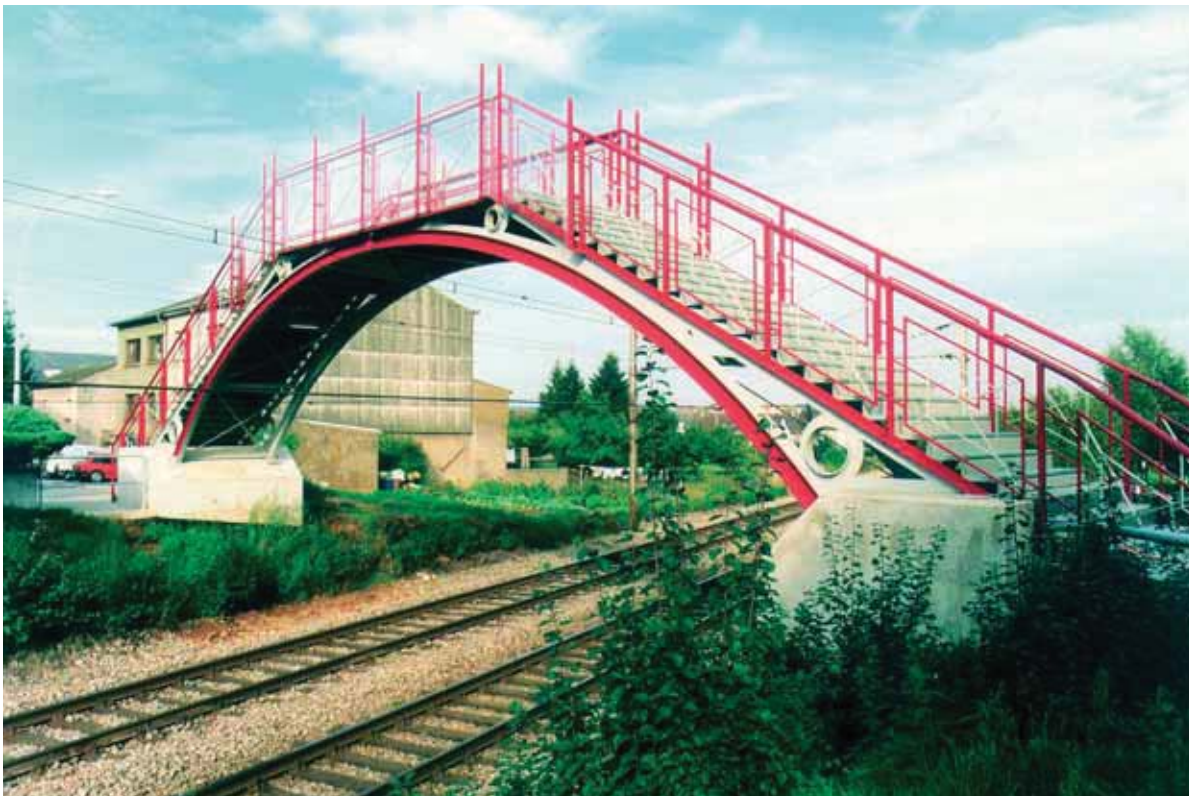
Footbridge near Schifflange, Luxembourg – Principle beams with an extreme curvature.
