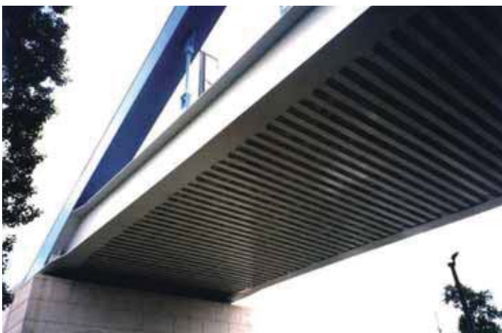
This example shows a bow-string bridge for the Mediterranean high speed railway line over the French highway A7 near Avignon (F). A filler beam deck has been used to span transversally to the bridge axis.
