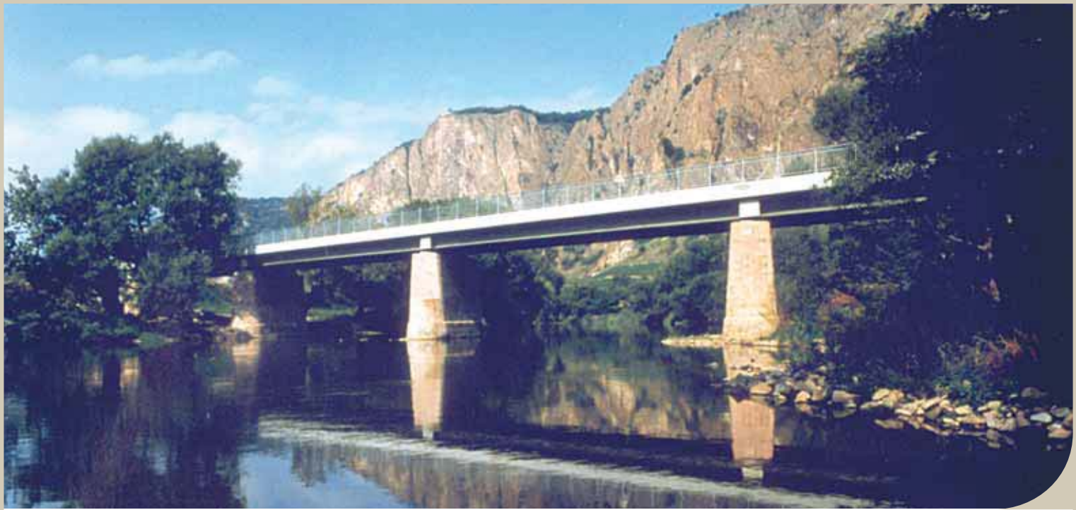
Reconstruction of bridge over the Nahe near Bad Münster am Stein, Germany – This bridge is located in a nature reserve. A composite deck was constructed on the existing piers.
