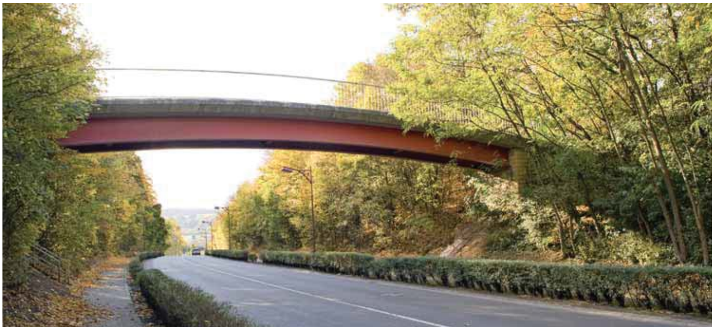
Footbridge over the national road at Wasserbillig, Luxembourg
