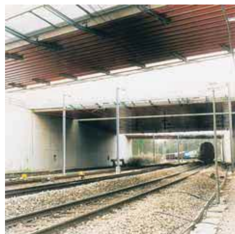
Filler beam bridge built over a heavy traffic railway line - High quality coating provides durable protection to lower flanges.
