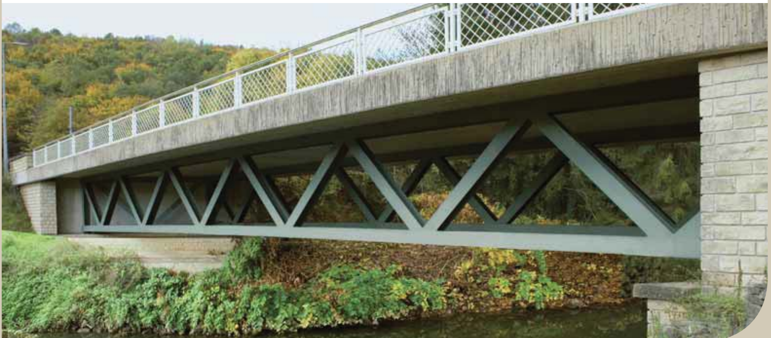
Costa Martina road bridge, Spain – Rolled beam truss girders, continuous over 3 span of 60.6 - 121.2 - 60.6 m. The picture shows the bridge before the erection of the precast slab elements on the upper chords.
