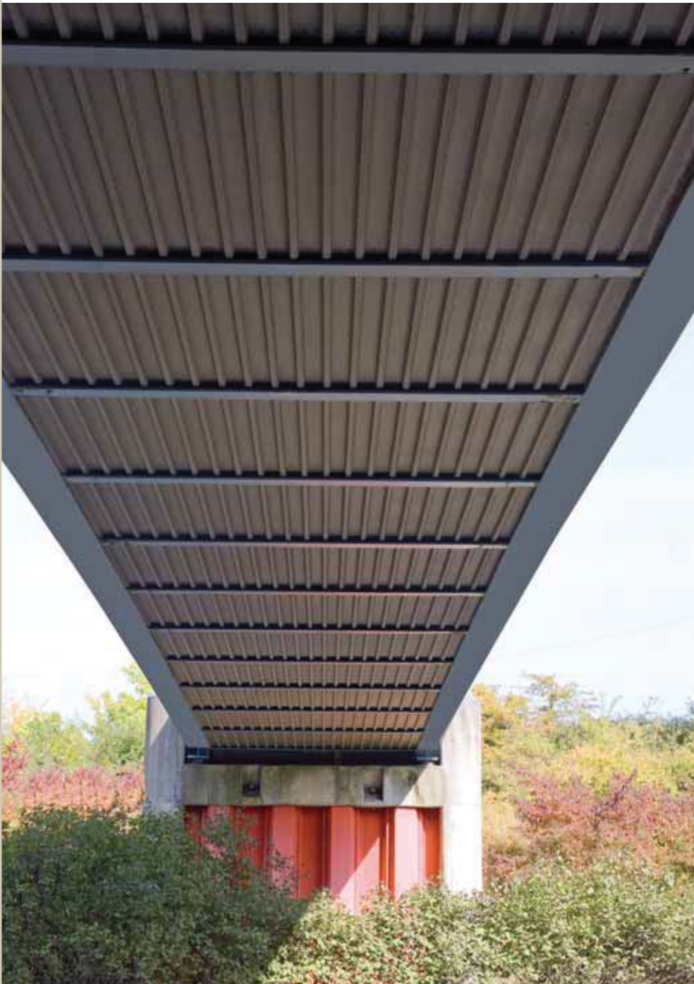
Bottom view on the footbridge at Soleuvre, Luxembourg – Sheet piles are used for the abutments.
