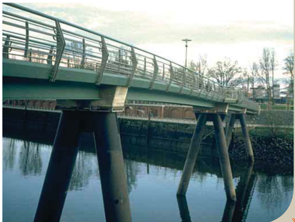
Footbridge over the Haken in Hamburg, Germany – Slender bridge with 4 spans of 25 m.
