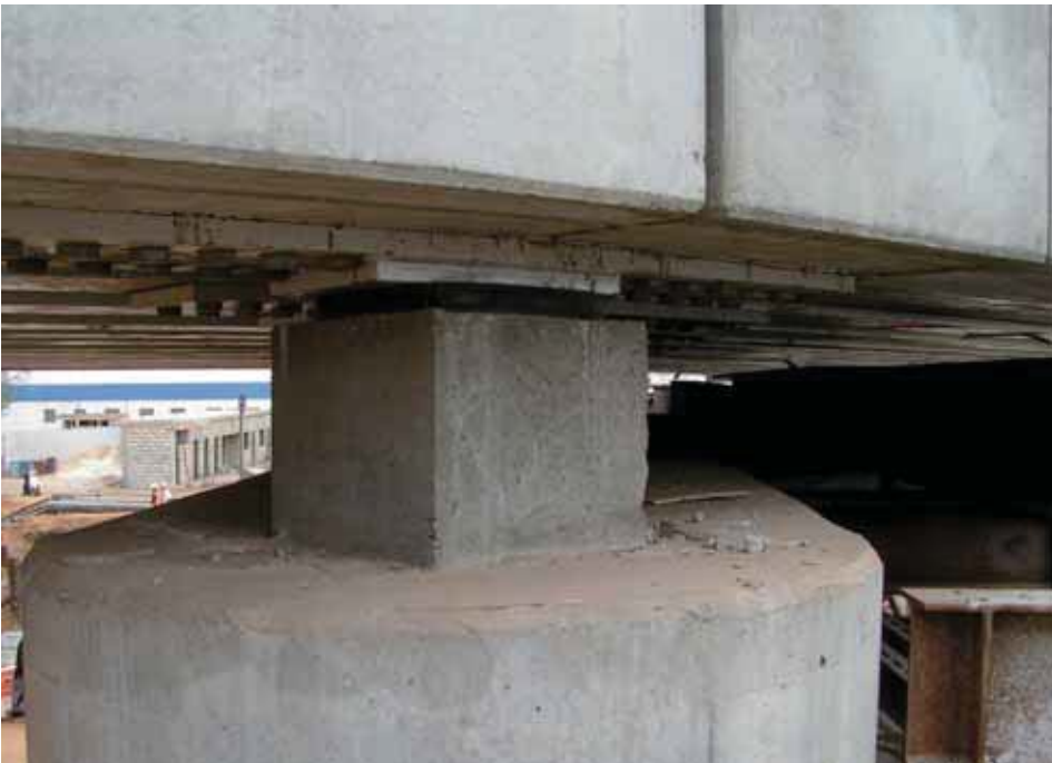
Pont de Cyrnos in Senegal - Detail of the support.
