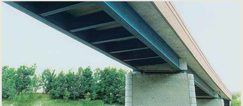
Railway bridge over the A23 motorway in Fretin, France - Four-span bridge with spans of 16.9 - 21.9 - 23.0 - 17.8 meters. The two continuous main girders and the bracings within spans are rolled beams; the cross beams at supports are made of reinforced concrete.
