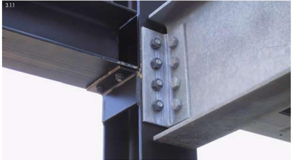
The steel bearing structure consists of vertical columns and horizontal beams, usually connected by bolting (pic. 3.1.1). The horizontal forces due to wind and braking of cars are transferred horizontally through the floor slabs to the vertical wind bracings or shear walls (e.g. stiff staircases).
