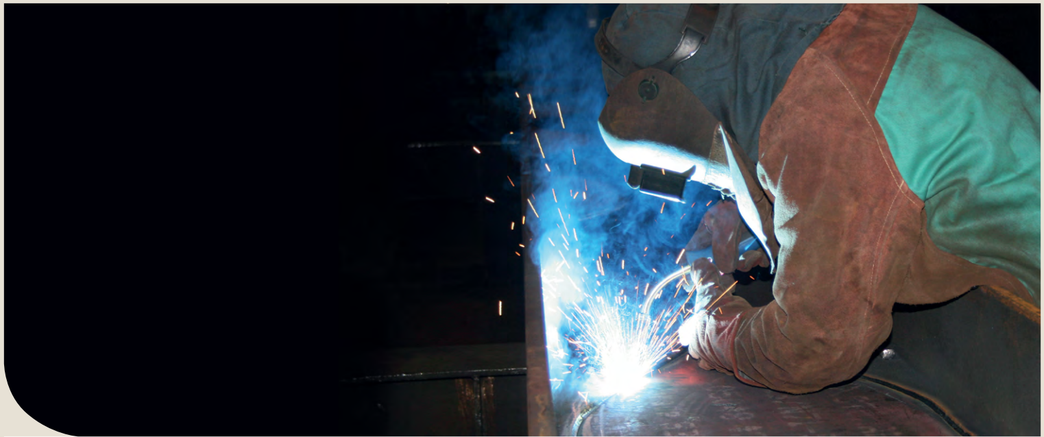
Figure 7: Fabrication of Angelina™ beams
