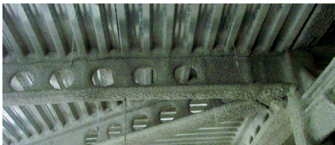
Figure 27: Protection by spraying on ACB® beam
