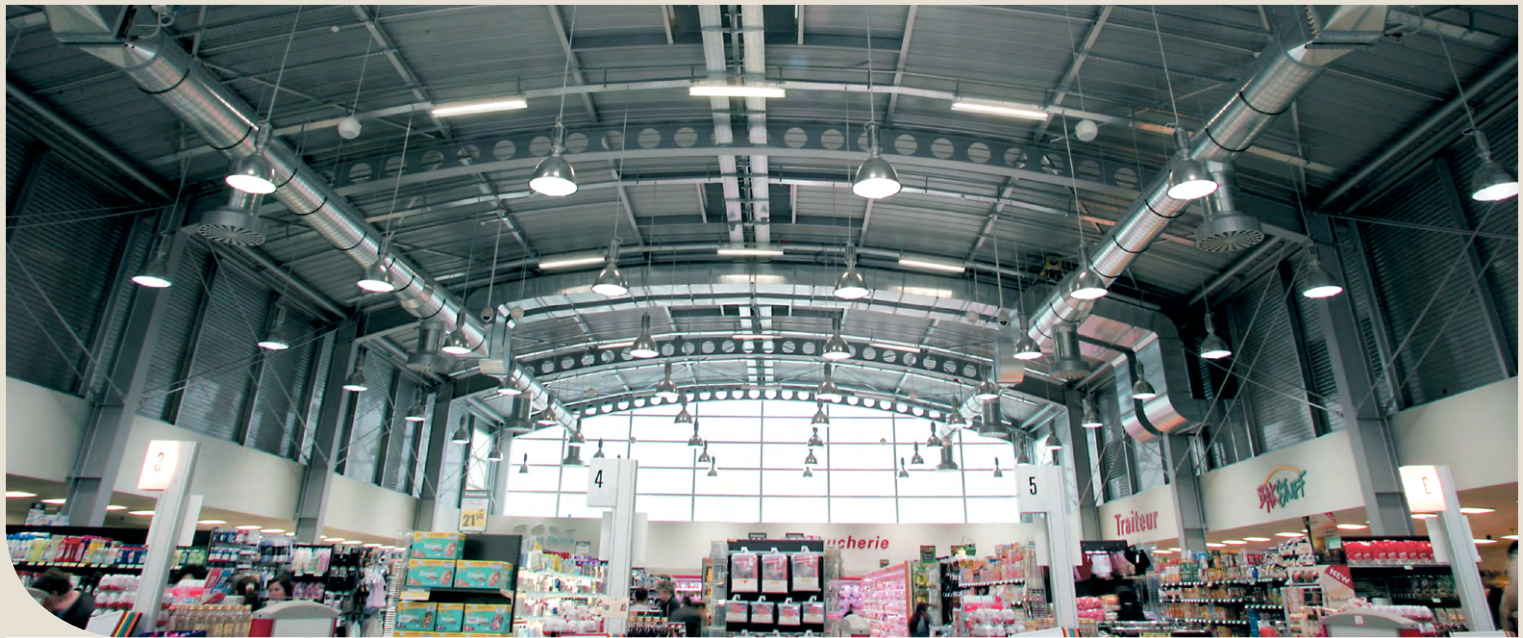
Castellated beams spanning 25 meters and featuring important camber
