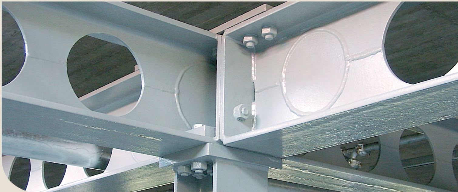
ACB® beam featuring filled openings at support
