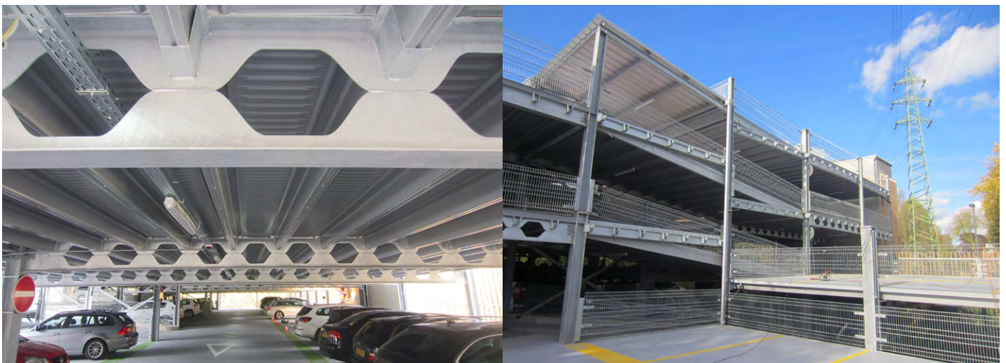
Figure 5: Castellated beams used in parking structures
