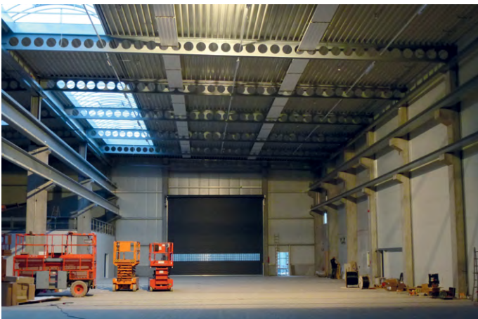
Figure 2: ACB® roof beams
