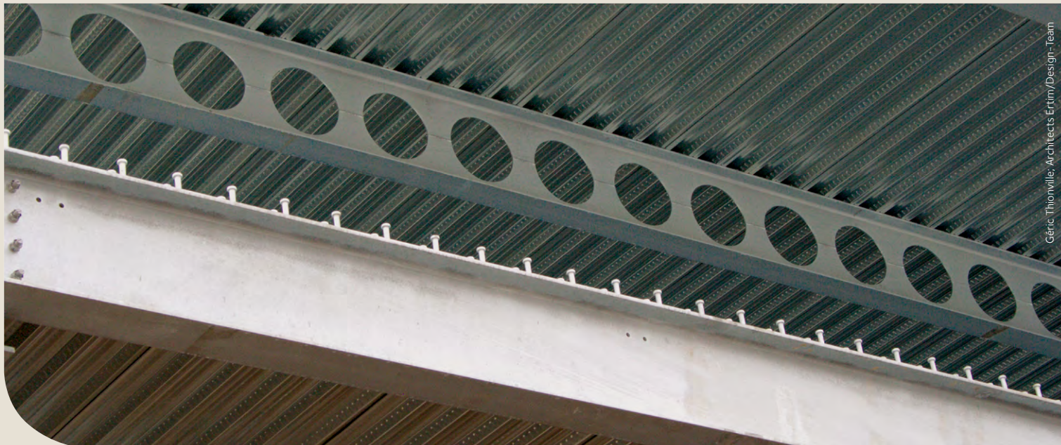
Figure 26: Composite floor beam
