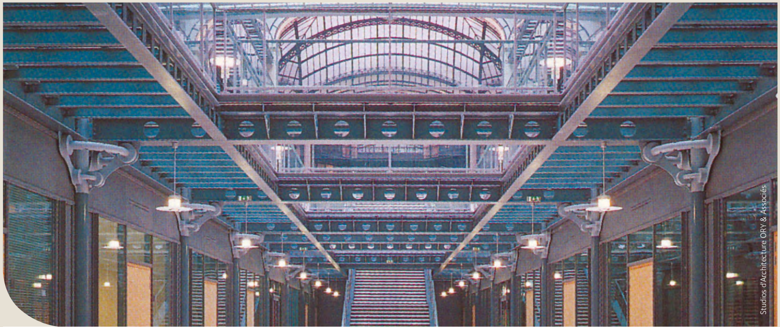
Figure 4: Renovation using ACB® beams at headquarters of Crédit Lyonnais, Paris
