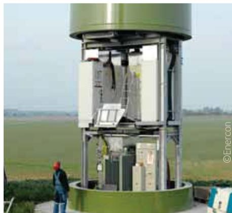
figure 8: Transformer and switch equipment
