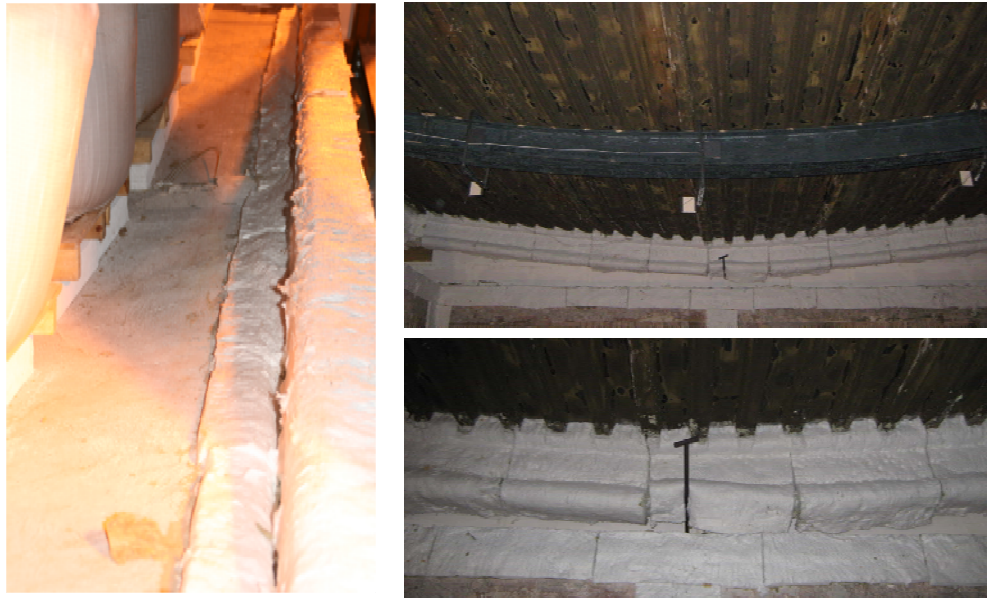
Figure 7.37 Collapse of edge beam
