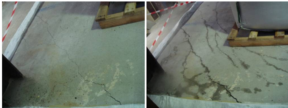
(a) At the beginning of fire test
