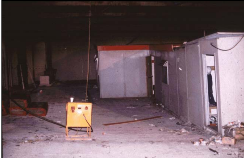
Figure 4.2 View of deformed floor above the fire (the maximum deflection was about 600 mm)
