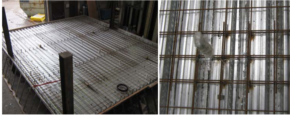
Figure 7.43 Overlapping of reinforcing steel mesh in composite slab
