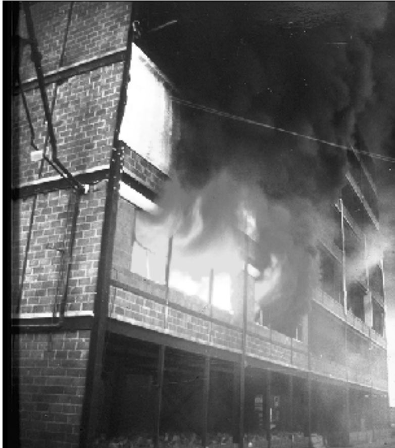
Figure 2.18 External view of fire
