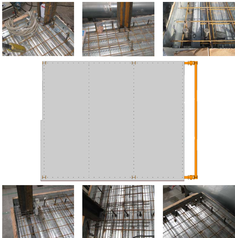
Figure 7.23 Different steel and concrete composite connection configurations
