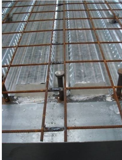
(a) Welded reinforcement joint prior to the concrete casting
