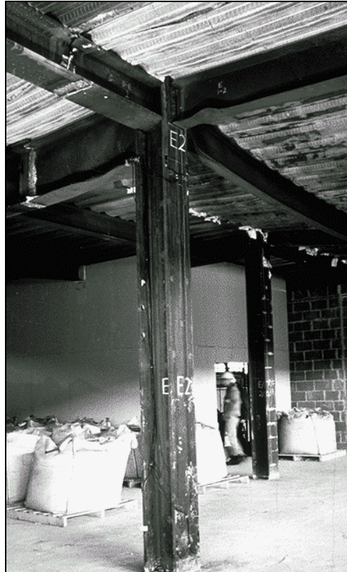
Figure 2.10 View of structure following test
