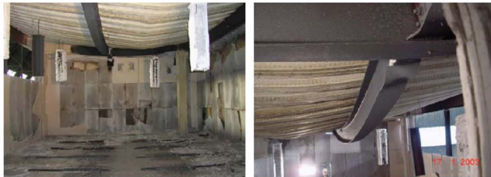
Figure 2.25 View of the floor after the test
